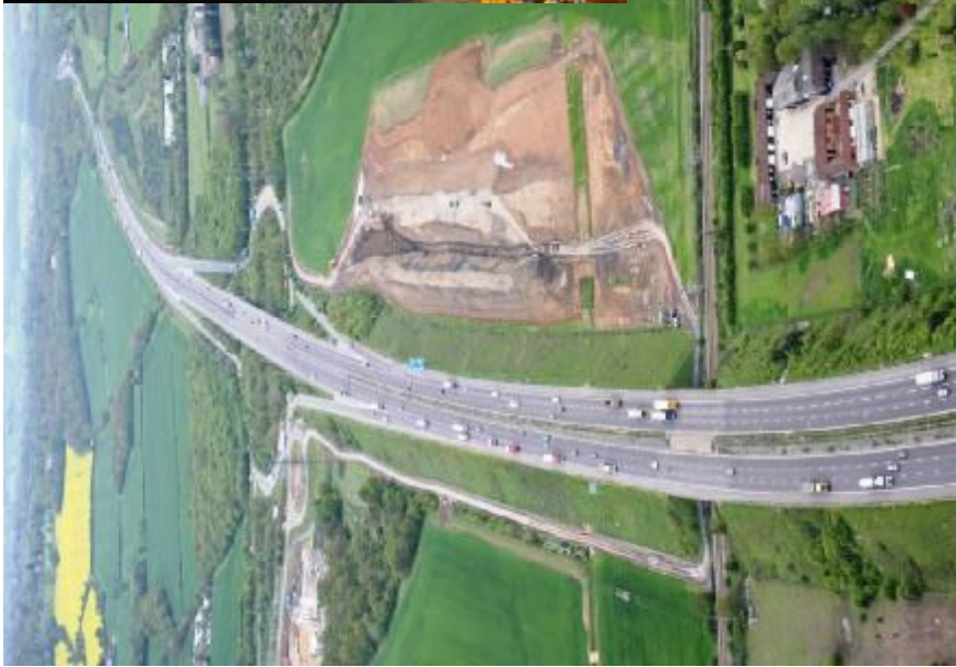
Upminster Bund under construction. This bund will finally be 4m above the carriageway and is to protect the residents of Cranham from the M25.
